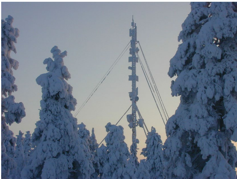
Military counter-intelligence acquires information on intelligence activities that threaten critical infrastructure or functions vital to society.
