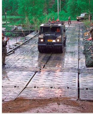
A pontoon bridge built by engineers.
